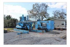
The sheeting machine gently pushes the iron sheeting into the ground with little to no vibration and very little noise.
