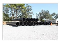
Rows of 54-inch HDPE pipe are stacked in the Safety Harbor laydown yard. These will be fused and pulled through the tunnel under the canal.
