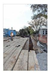
A row of the iron sheeting has been installed along the perimeter to shore up the area where the horizontal directional drill sending pit will be. In the foreground, what look like Paul Bunyon-size railroad ties are crane mats. These protect pipe underneath from the weight of the crane.
